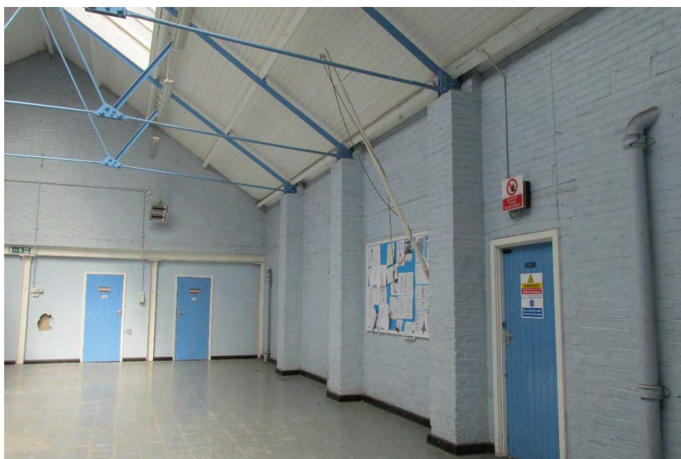
Figure 22: Eastern interior elevation, showing brick buttresses and earlier pipework, looking north
