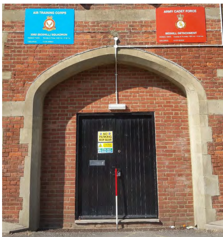
Figure 4: The filled-in earlier arch doorway, showing new brick entrance and modern smaller doors, looking north
