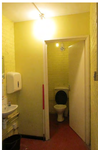
Figure 35: Individual toilet room in the older coal store, looking west
