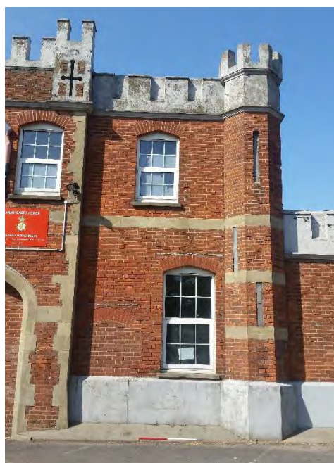
Figure 3: East octagonal tourelle tower, and modern window additions, looking north
