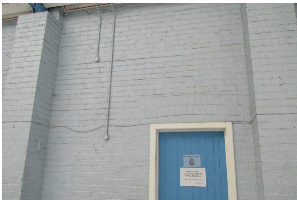
Figure 20: Detail showing beams above doorway on west wall, looking west
