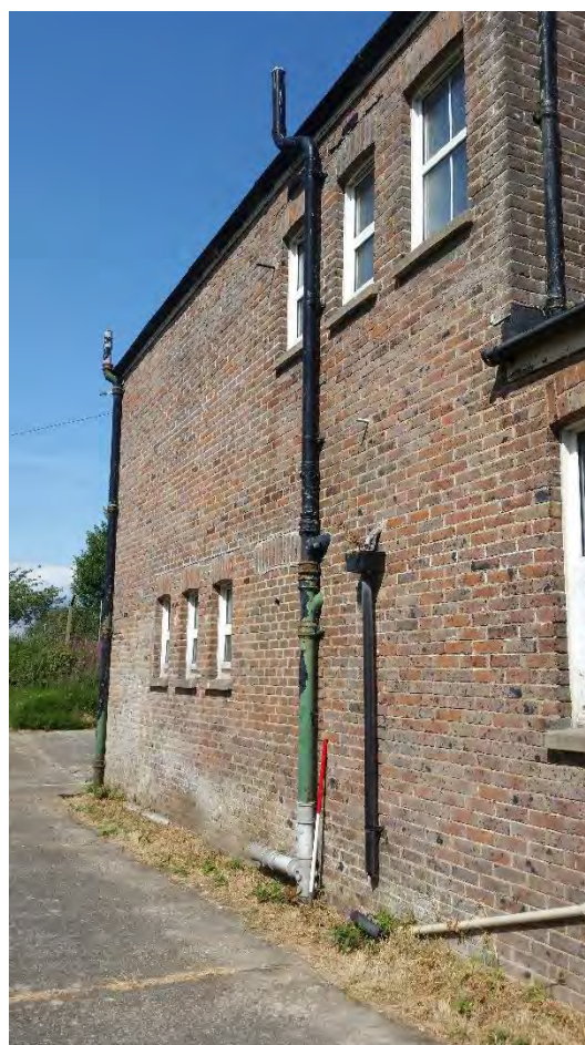
Figure 8: The rear of the drill hall, two-storey block, looking north east
