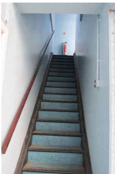
Figure 44: Original south east staircase, looking south
