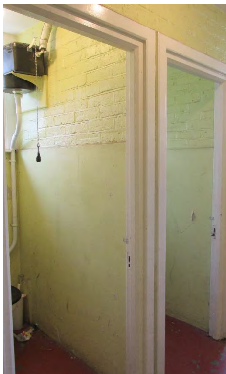
Figure 36: Toilet block, with door frames and concrete floor, looking north west
