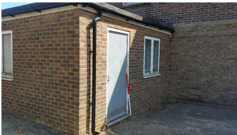
Figure 12: Modern square extension to rear elevation, looking south east
