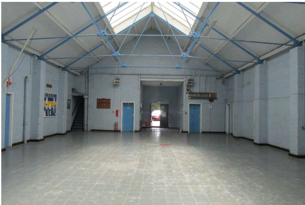
Figure 16: Main hall, showing entrance, looking south
