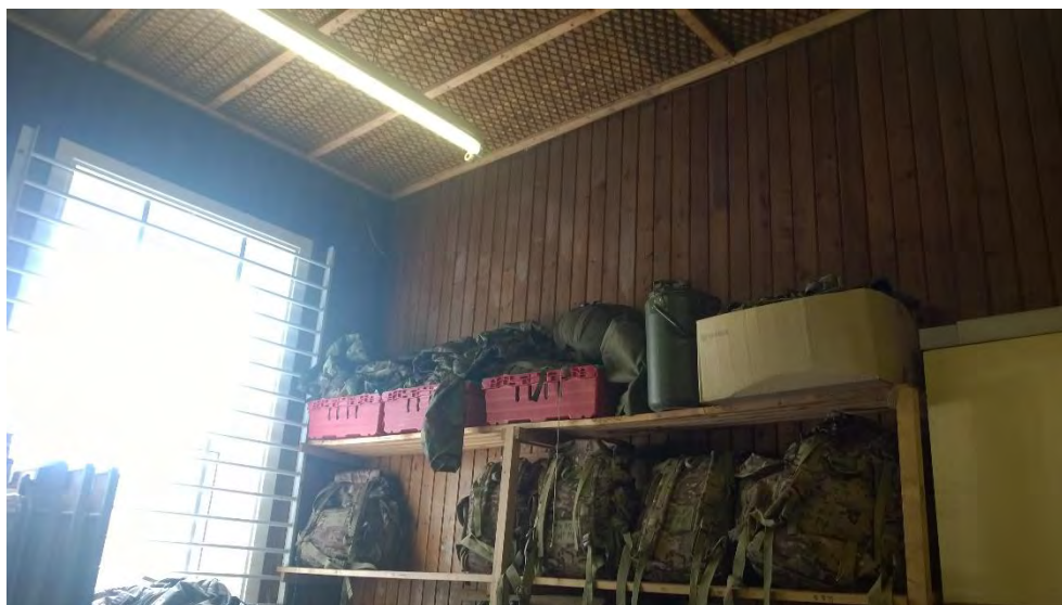
Figure 24: The panelled walls and ceiling of the store/saddle room
