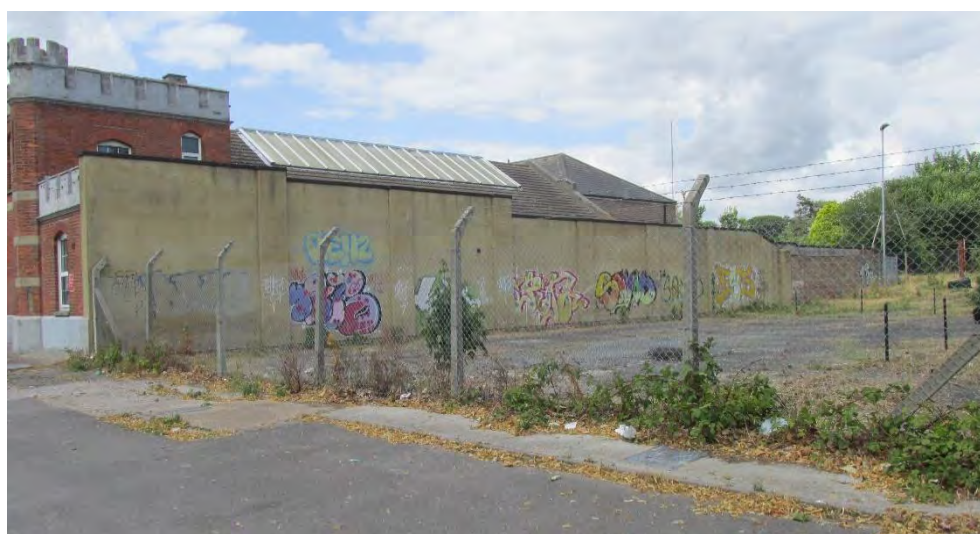
Figure 14: Eastern elevation of the 1914 drill hall, incorporating the west wall of the 1901 drill hall, looking north west
