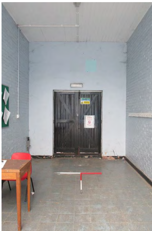
Figure 18: The entrance hallway showing the new doorway, and tiled floor, looking south
