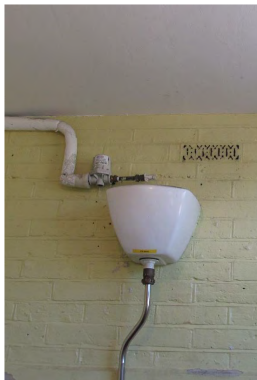
Figure 37: Original metal ventilation brick in urinal wall, looking west
