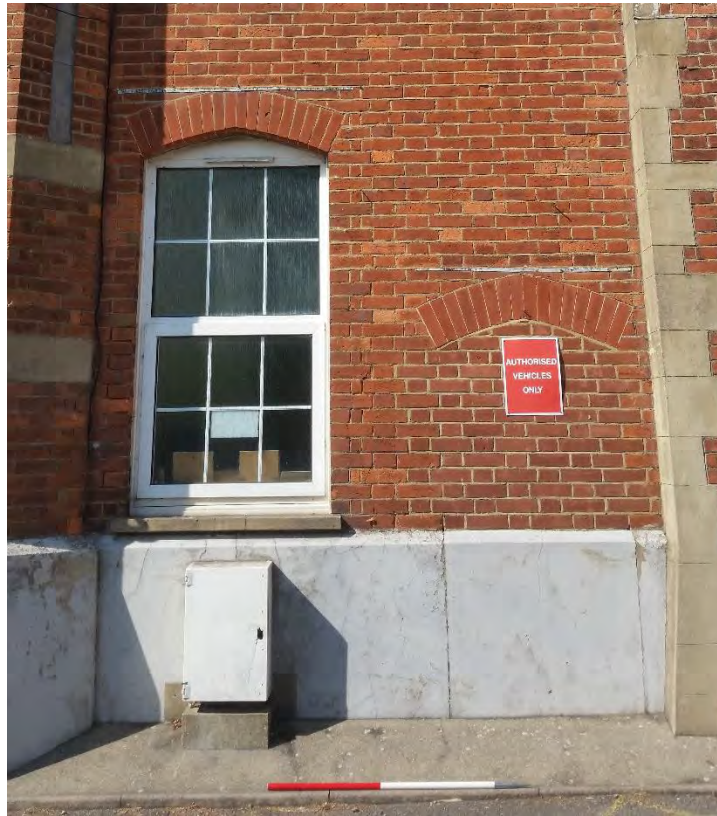
Figure 5: Filled-in smaller doorway on west of main entrance, looking north
