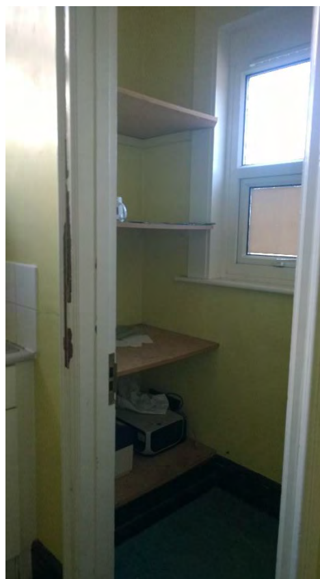
Figure 46: Earlier WC, used now as a cupboard, looking north east
