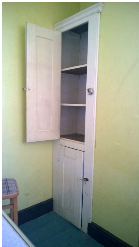
Figure 45: Original cupboard in first floor kitchen, looking south east
