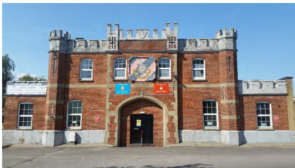
Figure 1: Principal elevation of the 1914 drill hall, facing north
