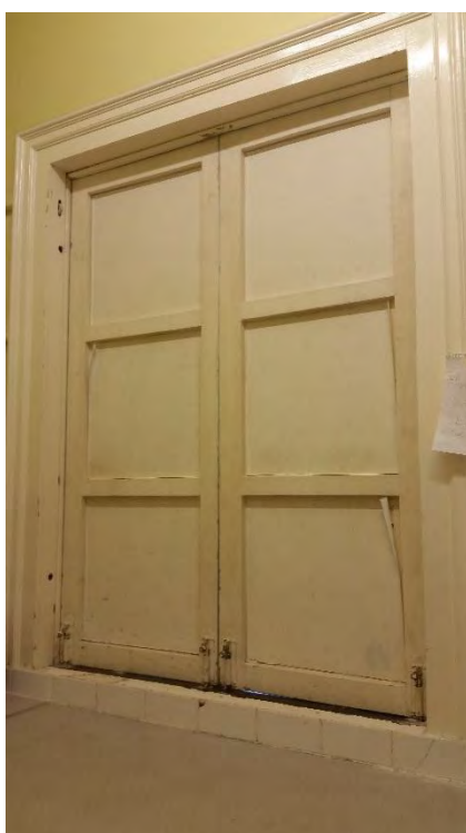
Figure 40: Serving hatch in kitchen still in use, looking west
