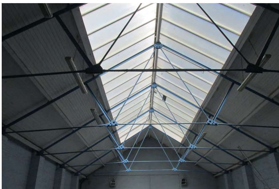
Figure 17: The roof trusses and roof lights, looking south
