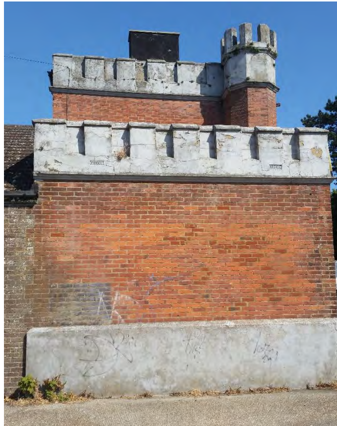
Figure 6: West elevation of main two-storey office block, looking east
