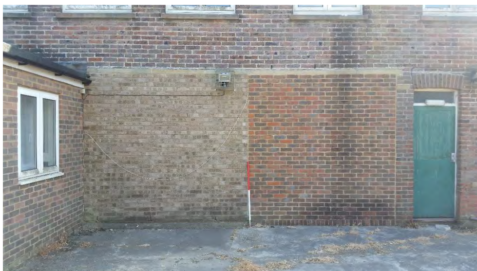
Figure 11: Filled-in earlier cart storage entrances, looking south
