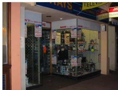
internal lattice shutters
