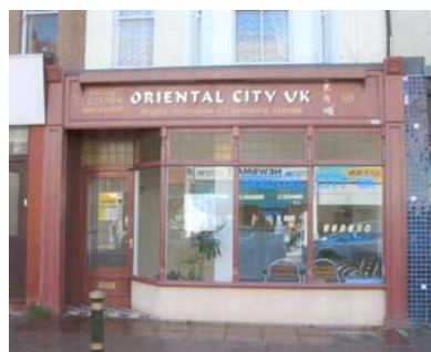
good modern shopfronts constructed in timber with traditional paint colours
