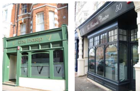
good modern shopfronts constructed in timber with traditional paint colours
