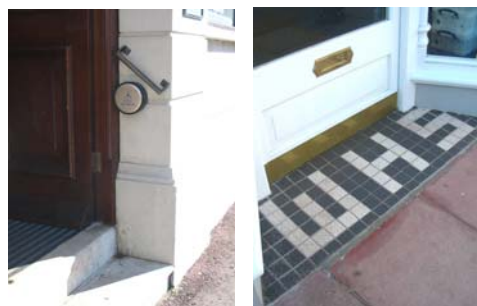
call button in a historic shopfront (left) and level entrance threshold in a new shopfront (right)
