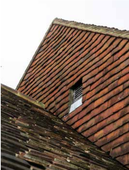
Details of a clay plaintile roof and a gable covered with hung clay tiles.
