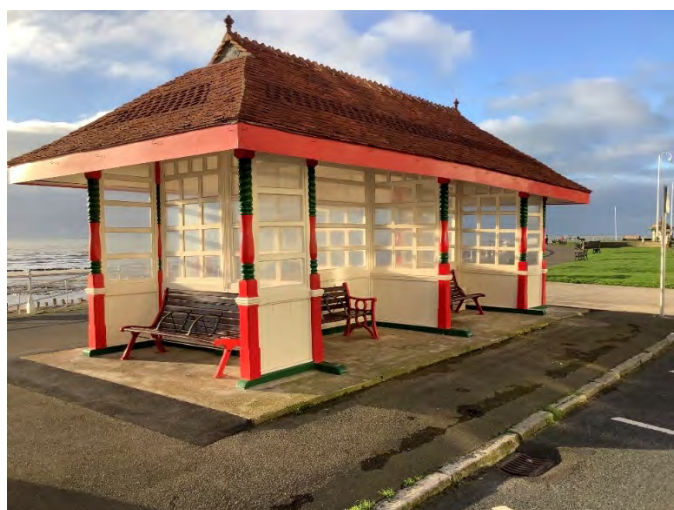
Bexhill Seafront Shelter refurbishment
