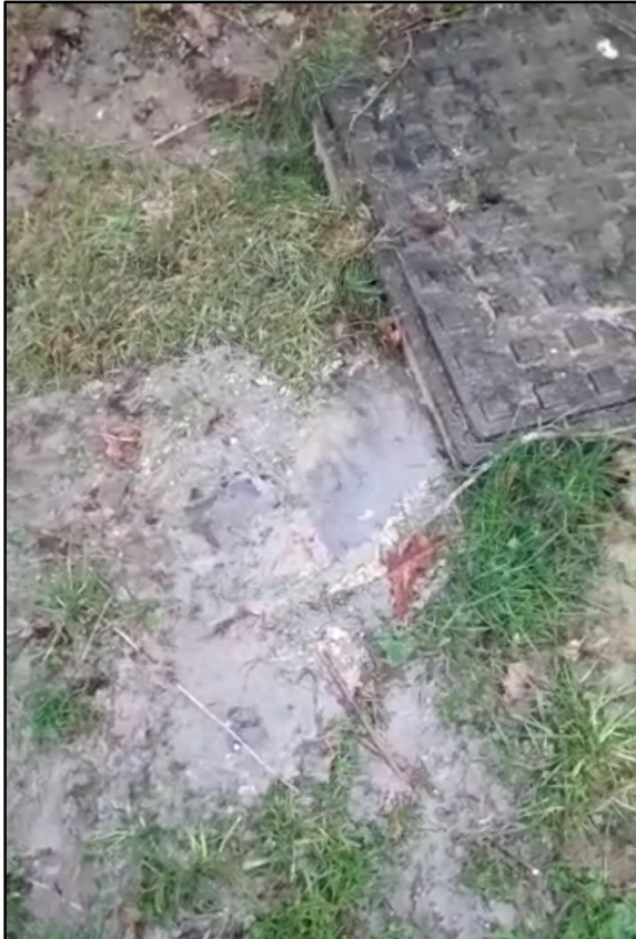
Frame grabs from cell phone videos of two separate incidents. On the left sewage is erupting from close to an inspection chamber. On the right sewage is gushing out with some considerable force from the underground sewage main.
