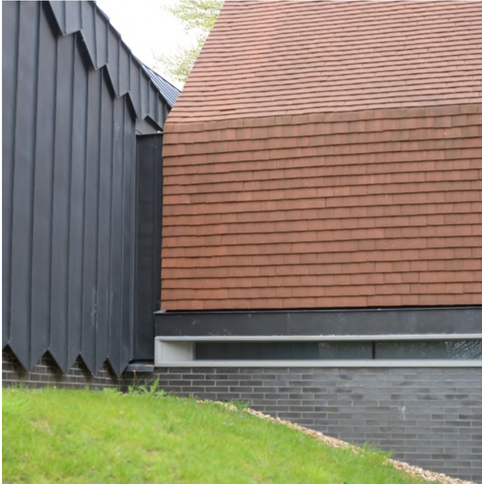
Above: Juxtaposing traditional and contemporary forms of materials with plain clay tiles and black patinated zinc. The Ditchling Museum by Adam Richards Architects. Image © Deeper Green
