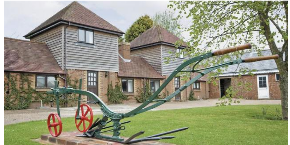
Above: New holiday lets at Park Farm, Crowhurst. The units are clustered around a courtyard in a manner reminiscent of a farmstead. Similar approaches in form and layout could be suitable for residential development. Image credit: Sonia Plato
