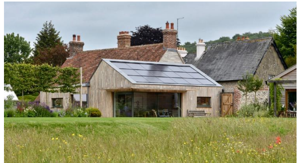
Above: A contemporary extension in a rural village. The additions are respectful to the context whilst exploiting opportunities for passive solar gain and an integrated solar roof (black finish). The cladding is Wealden-grown coppiced sweet chestnut. Image © Ian McKay / BBM Sustainable Design
