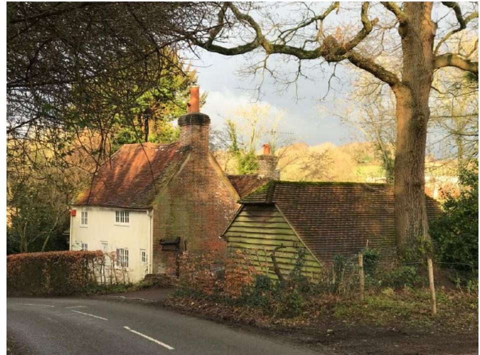
Above: Historic dwelling on Chapel Hill exemplifying the placement of buildings in a landscape dominated setting as well as some of the diverse cladding materials used traditionally in the Crowhurst context. Image credit: Deeper Green
