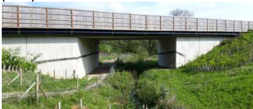
The 'dormouse bridge' underneath the carriageway (above)
