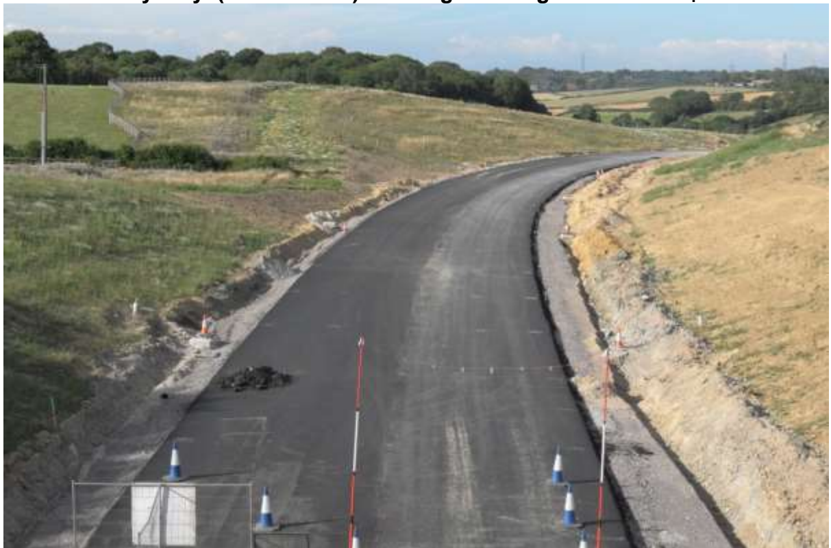
'Combe Valley Way' (TQ76311067) on bridge looking EAST 07 August 2015 Looking east
