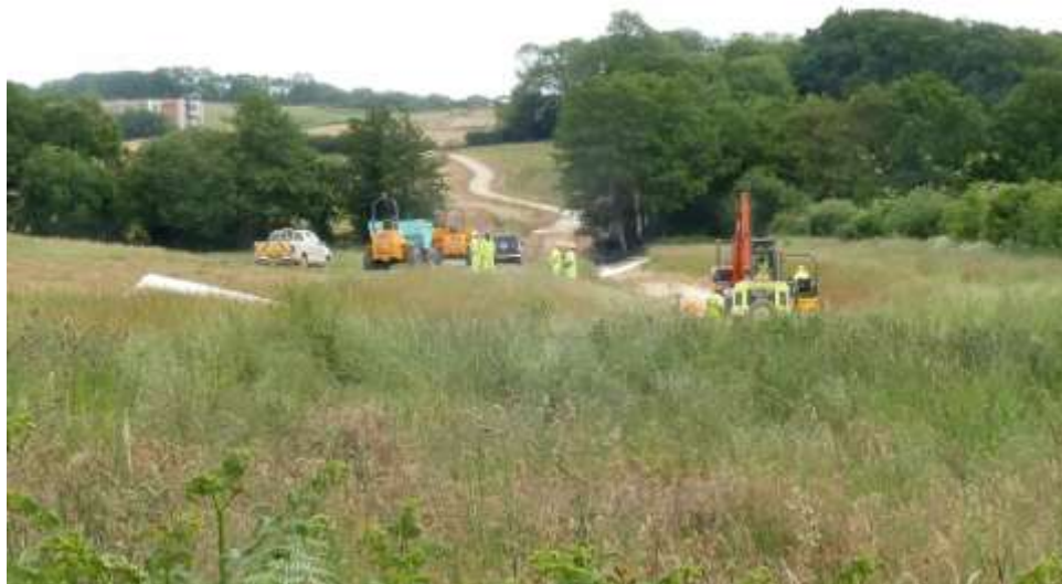
Greenway No.'Bexhill GrnWy/1' under construction. 18 January 2015
