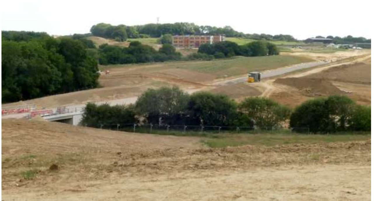
Combe Valley Way' (TQ76311067) on bridge looking WEST towards 18 Jan 2015
