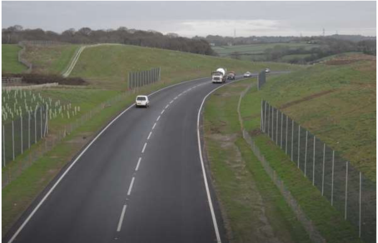
Combe Valley Way' (TQ76311067) on bridge looking east 21 Jan 2016
