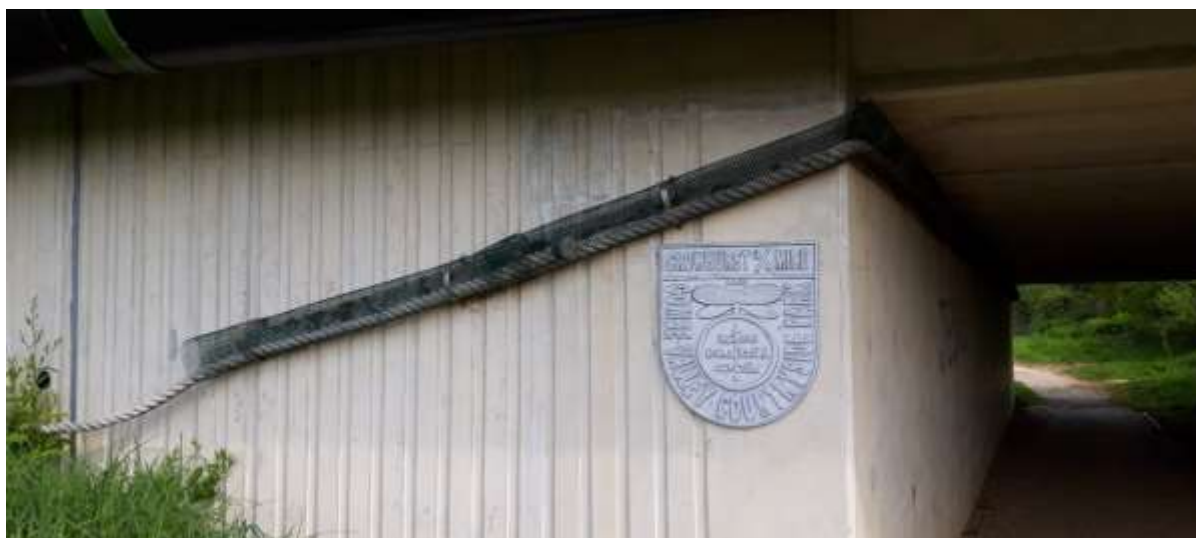
02 May 2019 The 'dormouse bridge' underneath the carriageway (above)
