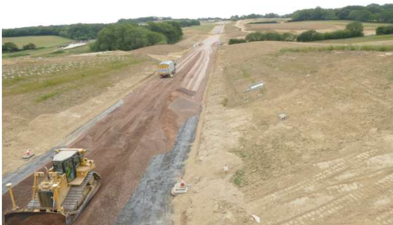
'Combe Valley Way' (TQ76311067) on bridge looking west, 2015
