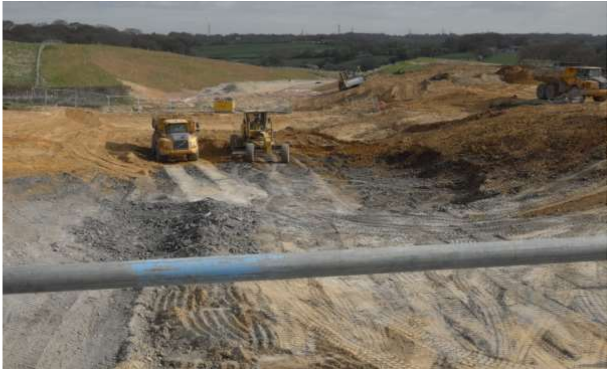
'Combe Valley Way' (TQ76311067) on bridge looking EAST 17 April 2015
