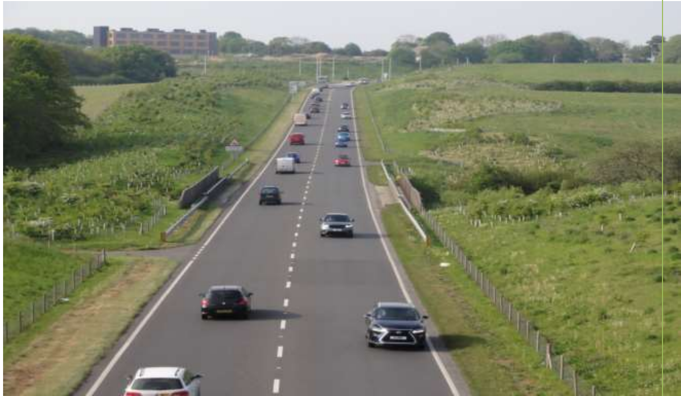
'Combe Valley Way' (TQ76311067) on bridge looking WEST
