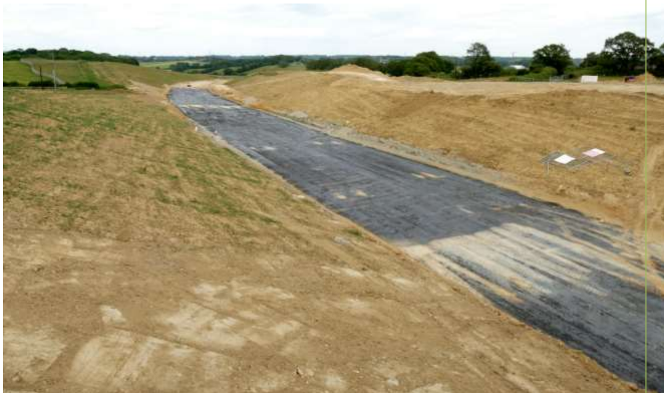
'Combe Valley Way' (TQ76311067) on bridge looking WEST
