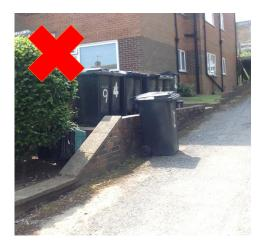
This is an example of a poorly designed storage point for a communal building which in this example is also the collection point. The containers sit above the vehicle access and are difficult to manoeuvre to the collection vehicle. The bins have to be bumped up and down a step and taken out and put back one at a time. It is also very difficult for residents to gain access to their bin to dispose of waste.
