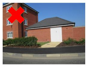
This development has got everything right in terms of providing a good storage area, but it is inappropriate due to the lack of a dropped kerb to manoeuvre bins over. This is a significant error as this bin stores houses large 1100 litre bins which should not be required to be moved over distances to the nearest drop kerb (safe manual handling) or will be damaged if alternately bumping up and down over the kerb on a regular basis.
