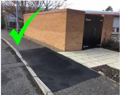
An excellent example of an appropriately located and designed communal bin store. The store is enclosed, secure, with a smooth flat surface for manoeuvring bins, with a dropped kerb.
