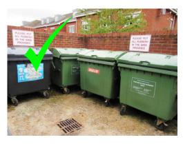
This is a good example where a durable bin store area has been built with consideration for drainage as it is an open air site. The floor surface is flat and hard wearing and there is sufficient space for the number of bins required and to manoeuvre them easily to the collection vehicle. In this example signage has been included to inform residents to make sure all waste is contained within bins.
