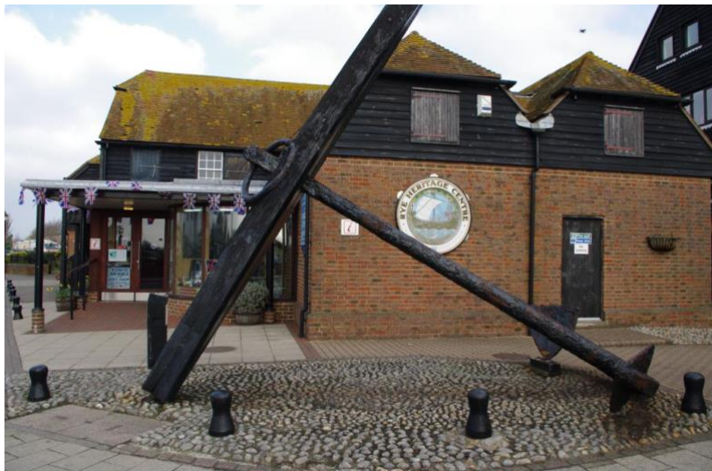
Figure 15: Rye Heritage Centre
